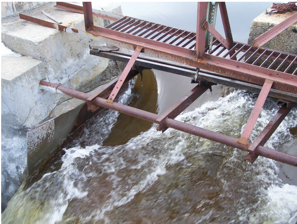
Water flows during High water conditions 11/07
