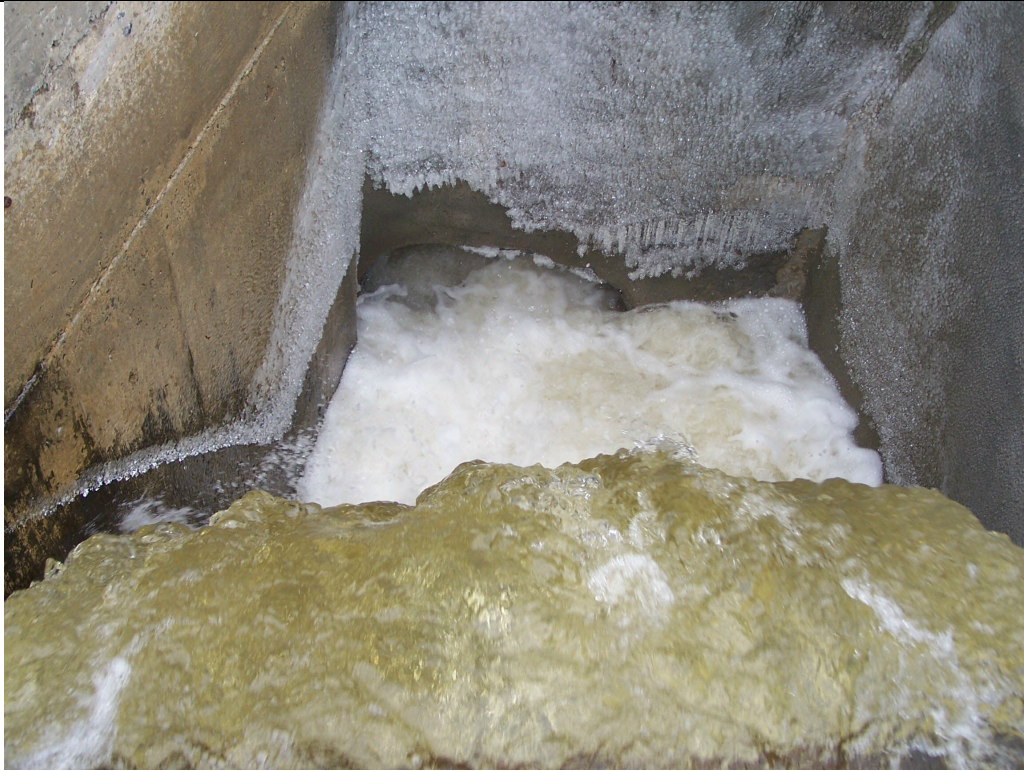
Box Culvert during High water conditions 11/07
