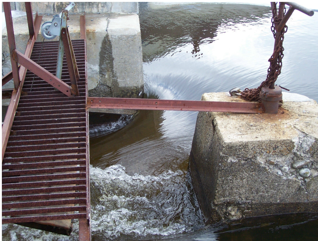
In flow of the MCA Dam 11/07
