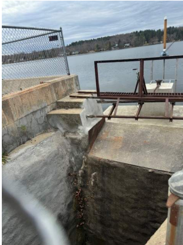
Completed repair work
