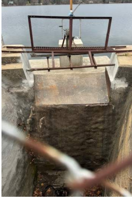
Completed repair work
