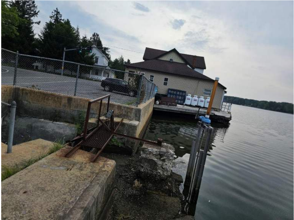
Abandoned Low Level Outlet Structure with Face Mounted Gate Frame and Cracked Concrete Structure
