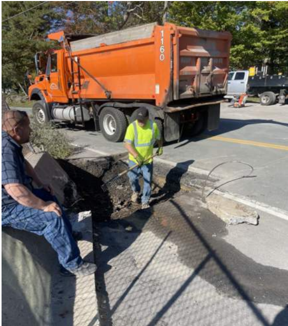
Repairs made by Schenectady County
