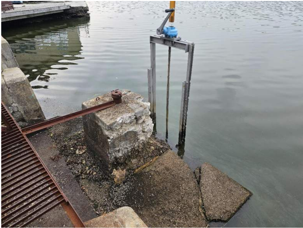
Abandoned Low Level Outlet Structure with Face Mounted Gate Frame and Cracked Concrete Structure
