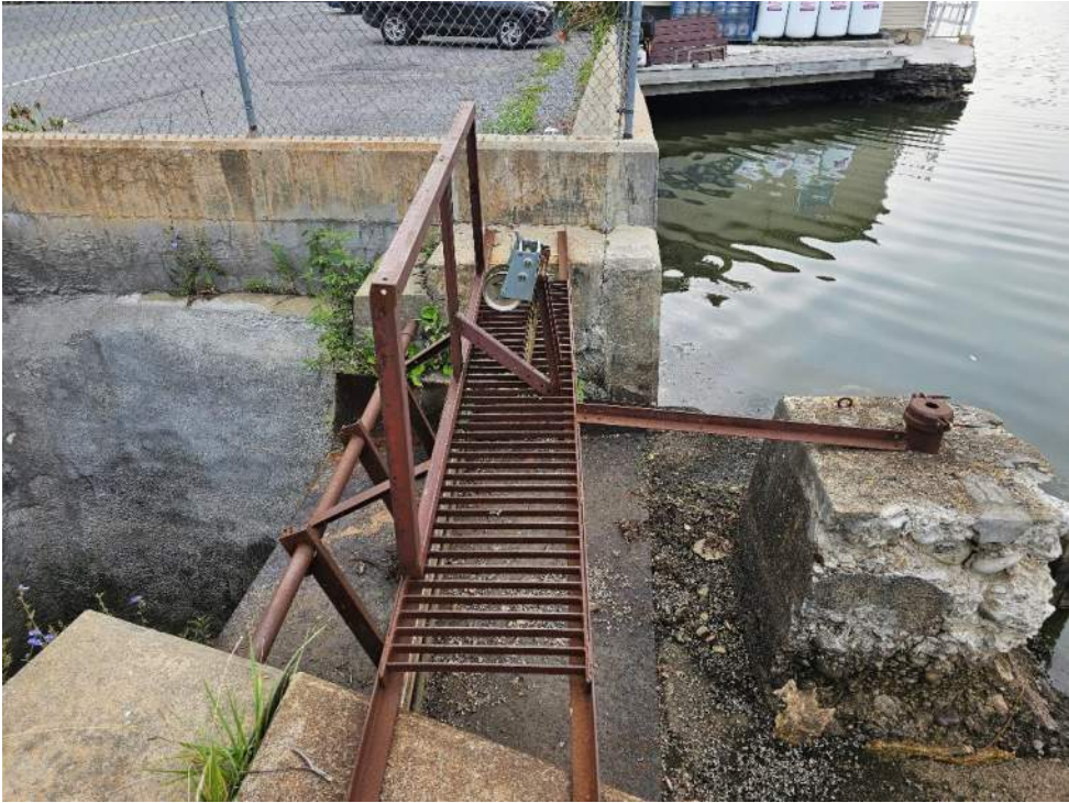
Spillway/Headworks Looking East
