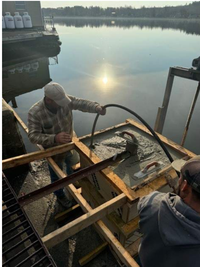
New concrete pour around abandoned low level outlet valve
