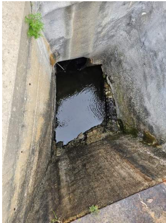
Upstream Face of Drop Inlet
