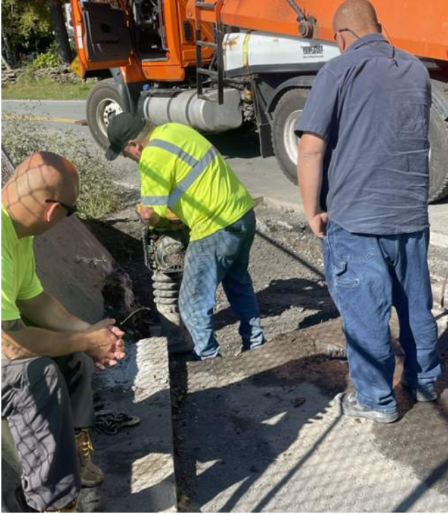
Repairs made by Schenectady County
