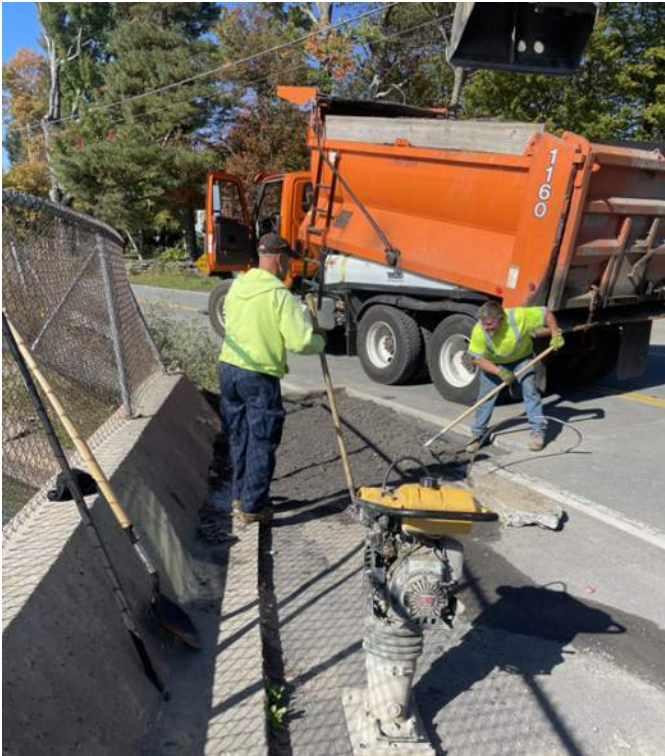
Repairs made by Schenectady County
