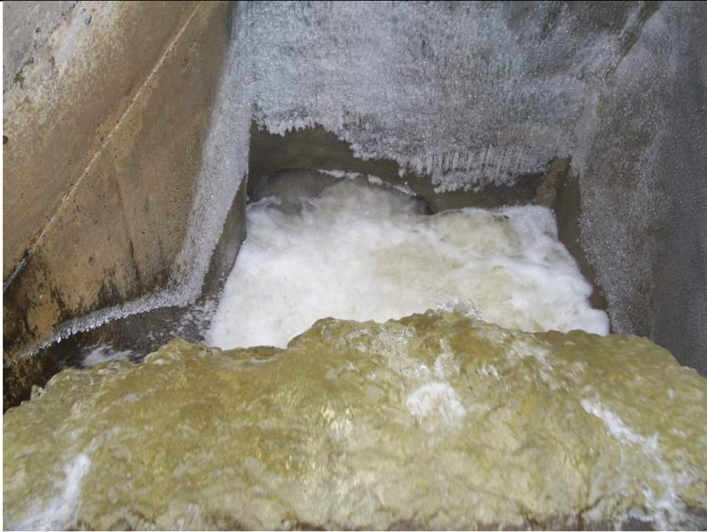
Box Culvert during High water conditions 11/07
