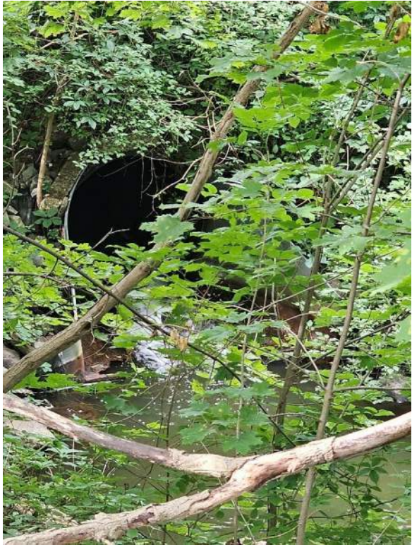
Outlet Pipe Looking South
