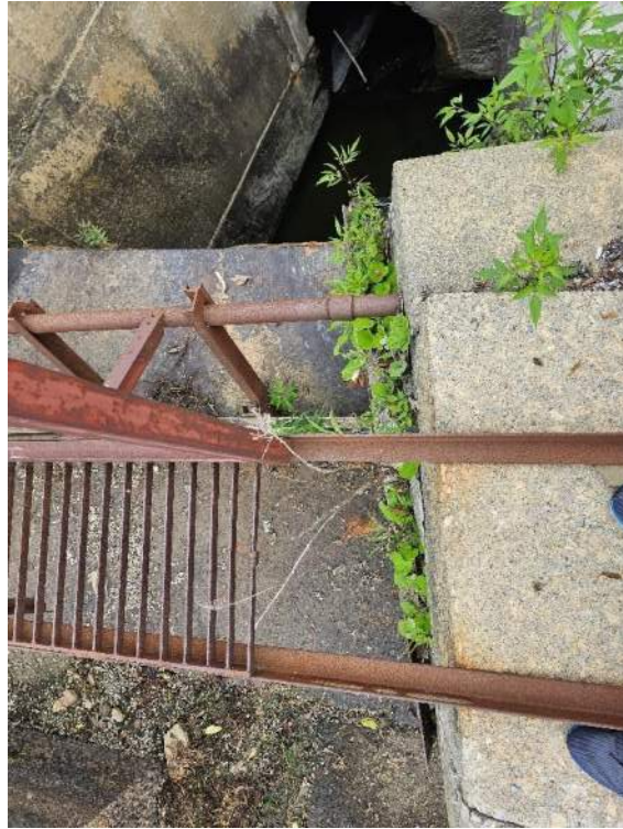
Metal Plate At Spillway Wall
