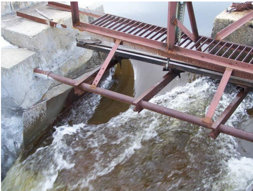
Water flows during High water conditions 11/07
