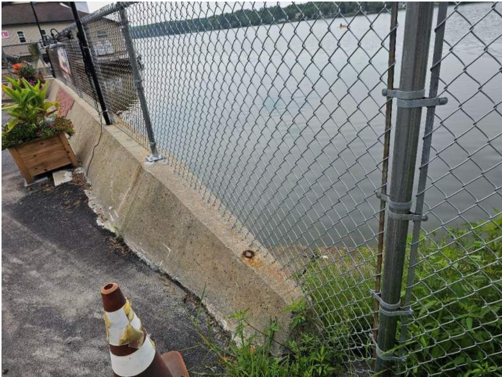
Back of Headwall, Looking East
