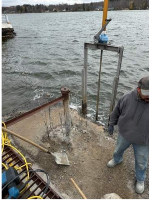
Demolished concrete around abandoned low level outlet valve
