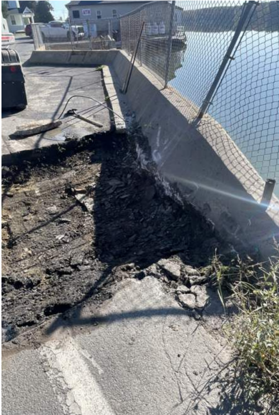
Schenectady County began repair work on 10/4/23
