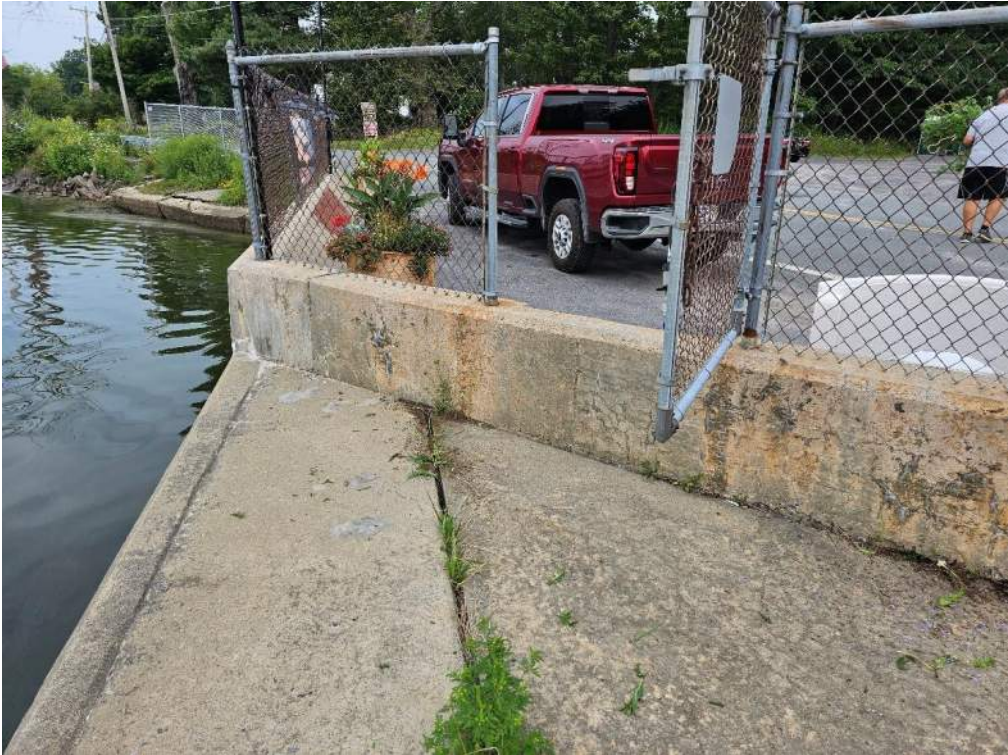
Auxiliary Spillway Looking West
