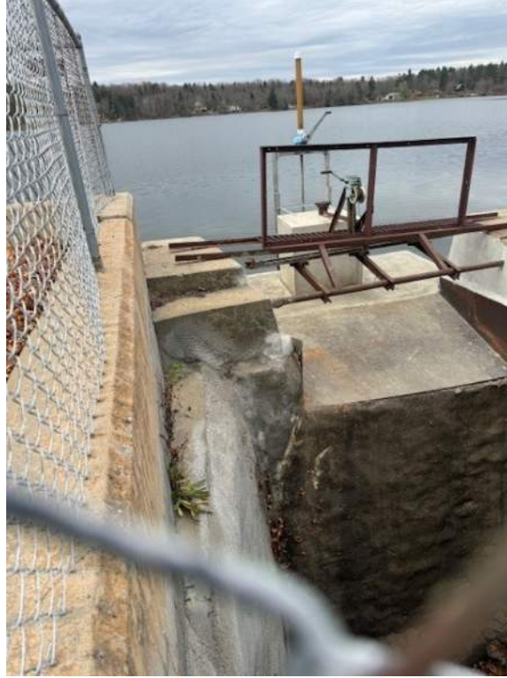
Completed repair work
