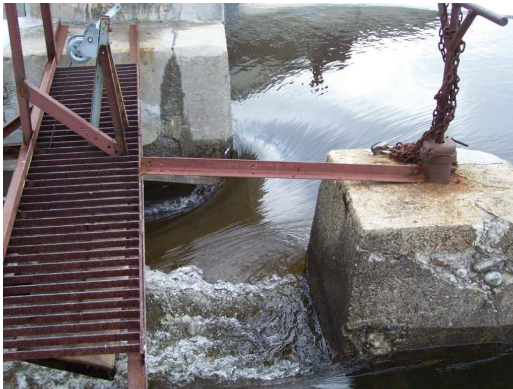
In flow of the MCA Dam 11/07
