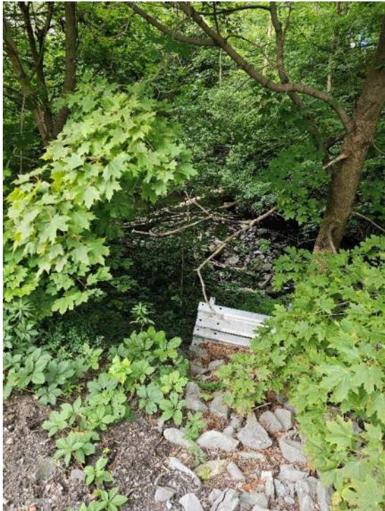
Outlet Channel Looking West
