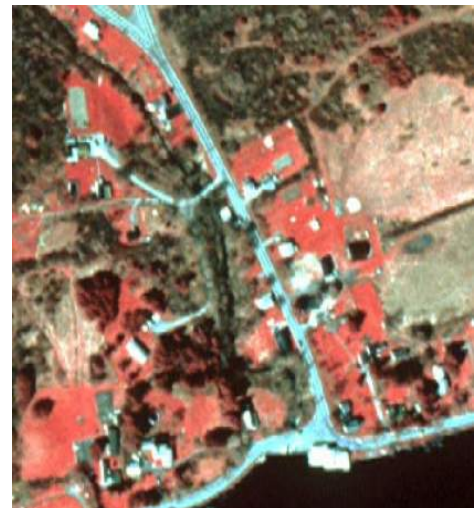
Mariaville Lake Dam
