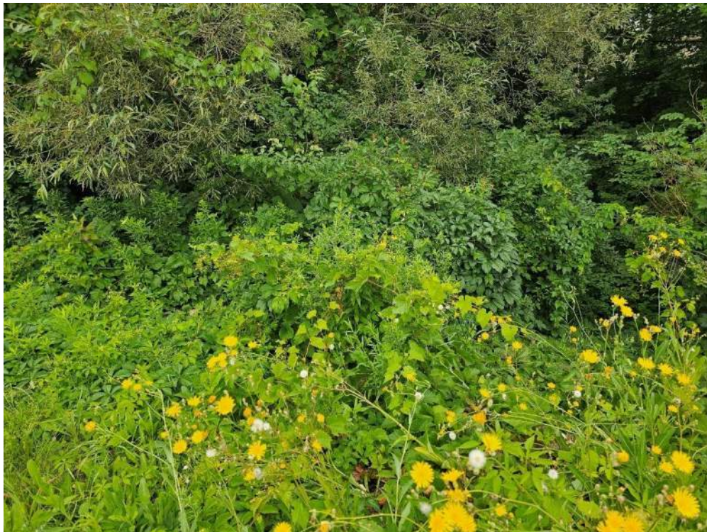
Downstream Embankment Looking North
