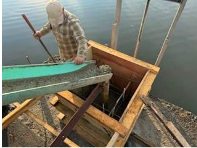
New concrete pour around abandoned low level outlet valve
