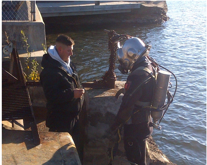
Picture above shows Diver from Seaway Dive Services on the November 4,2013 MCA Dam Dive
