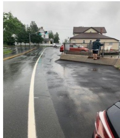
Completed roadwork Infront of our Dam with proper drainage
