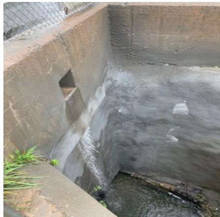
Newly Shot created repaired spillway
