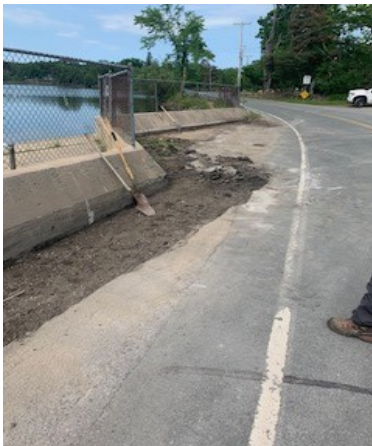
Road work on being Completed by Schenectady County DPW
