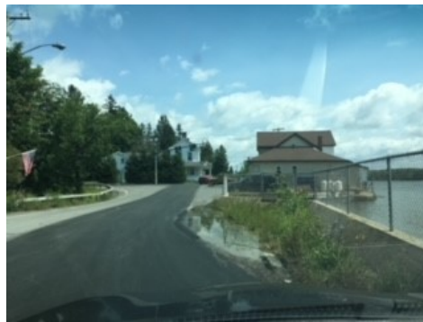
Roadway overgrown and muddy by Dam
