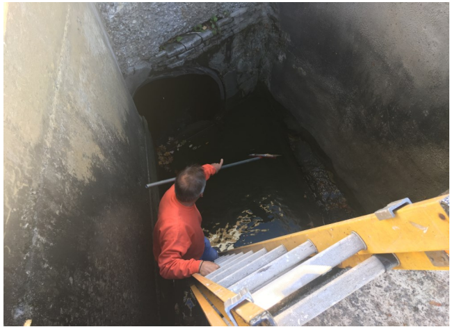
Chris Shaver working on the dam down the spillway 2017
